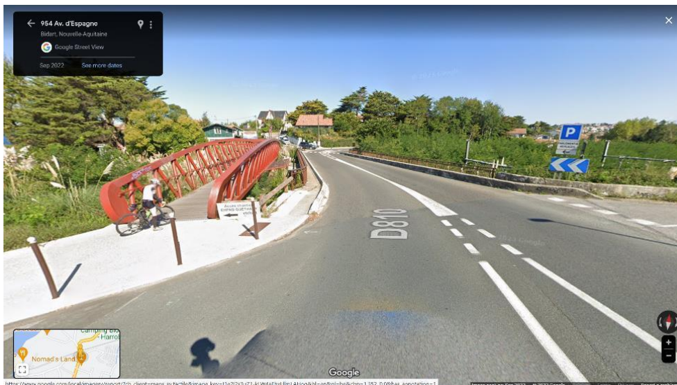
A new pedestrian and cycle bridge between Bidart and Guethary enables safe crossing of a TEN-T railway
