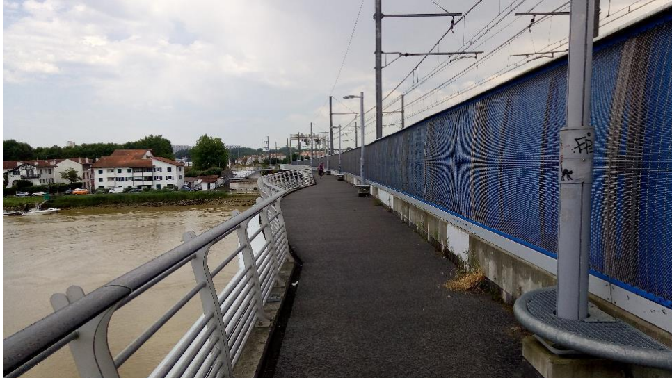
Charles-Vaillant bridge in Bayonne, combining TEN-T railway with cycle and pedestrian track.
